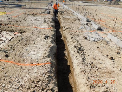
Underground sanitary being installed along the main corridor of Unit B
