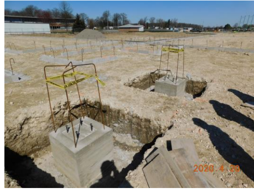
Columns installed in the main hub of the classroom wings
