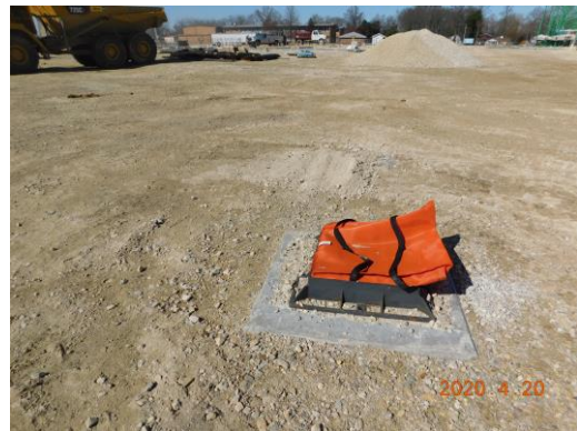
Site storm completed and protected East of the building
