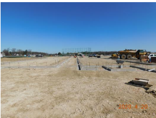
View from classroom hub looking North towards Unit B
