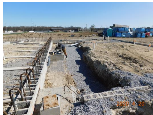
Pit dug and prepped for underground electric in main electrical room
