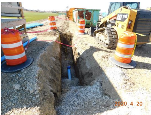
Water line installation East of the new building
