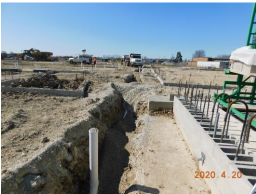
Underground plumbing to the east of the gym
