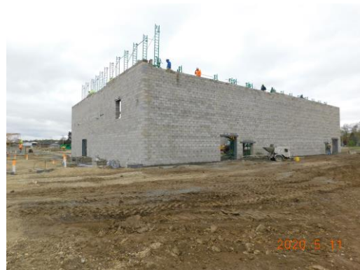
Gym walls from the North side
