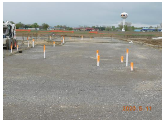
Sanitary stub ups in the classroom wing
