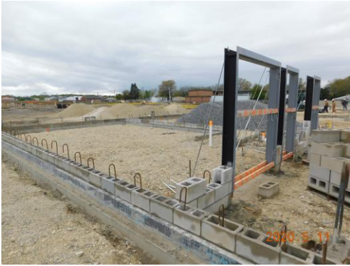
Doorframes off the stage area, east side
