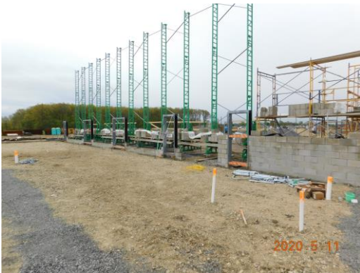
Doorframes and CMU installation on wall between kitchen and student dining
