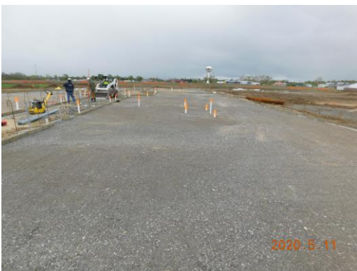
Stone pad prep for future concrete pours
