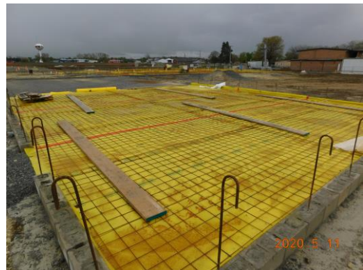
Floor prep for concrete pours in unit B
