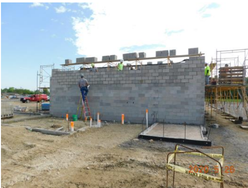
Unit D precast area CMU installation
