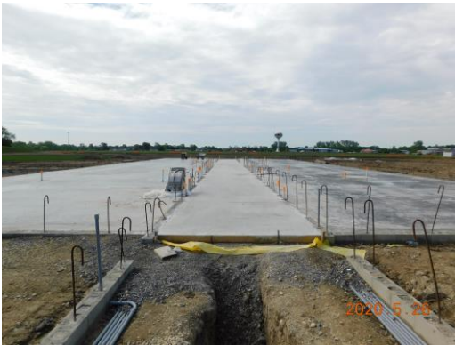
Concrete floor pours in Unit E
