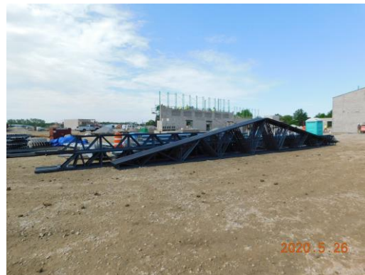
Steel trusses on site ready for installation
