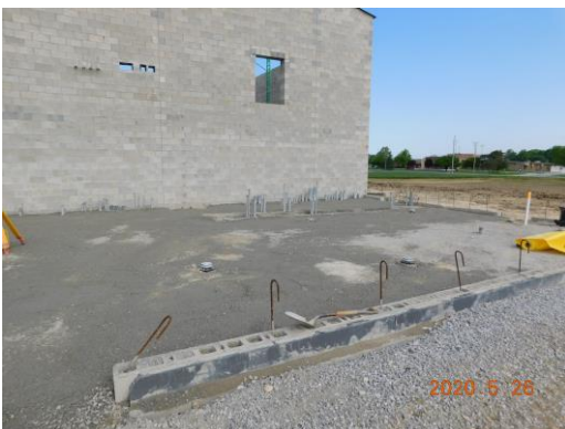
Floor prep in Unit A main electric room
