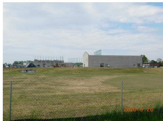
View of the building from the North side of the property
