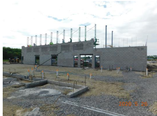
CMU wall installation between kitchen and dining
