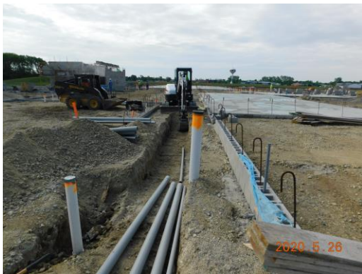
Underground electric installation down main corridor of Unit B
