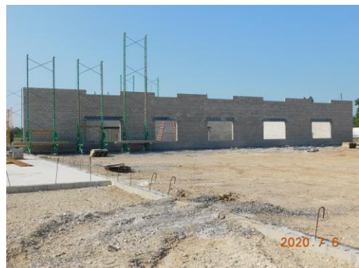
Unit C 1 st floor north exterior wall completed
