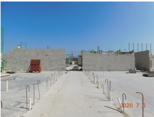
Unit C classroom hub CMU wall installation looking from Unit E
