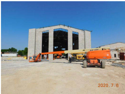
East side of student dining CMU wall completed
