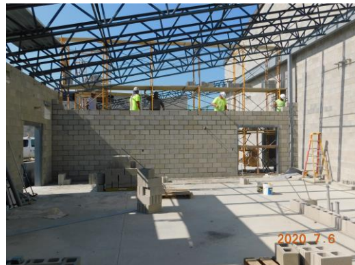
Unit A CMU installation at main electric room
