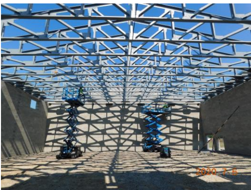
Gym trusses in place and detailing started
