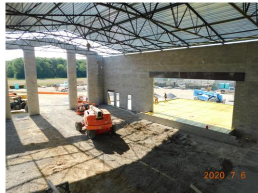
View inside student dining from the mezzanine
