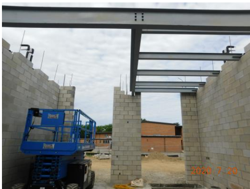
Steel installation around the stairwell in Unit C
