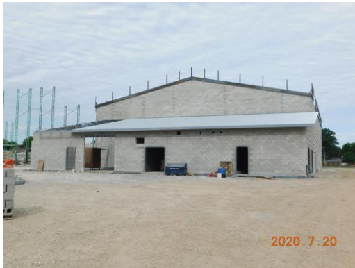
Roof decking being installed on the low roof of Unit A
