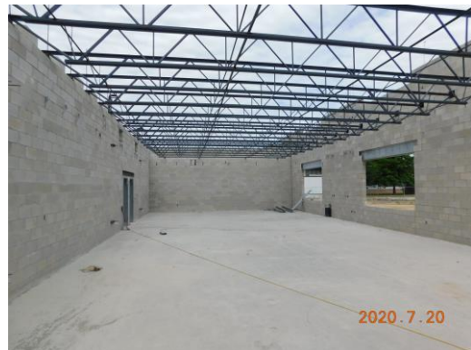
Bar joist installation in Unit C
