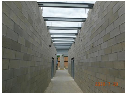
Steel installation in the corridor of Unit C
