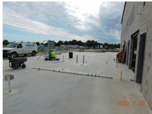
Kitchen floor has been poured
