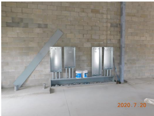
Electrical panel installation has started in Unit A
