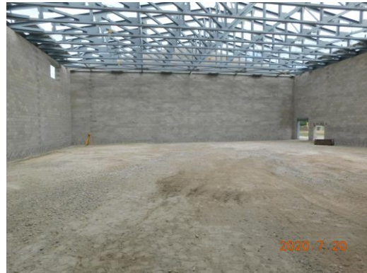
Gym stone grade being worked on in preparation for floor pour
