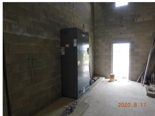
Switch gear installation has started
