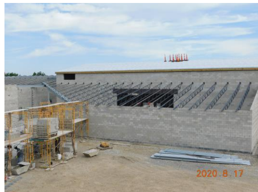
Steel joists over the stage area
