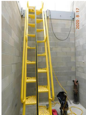
Stair installation to the Unit A mechanical mezzanine
