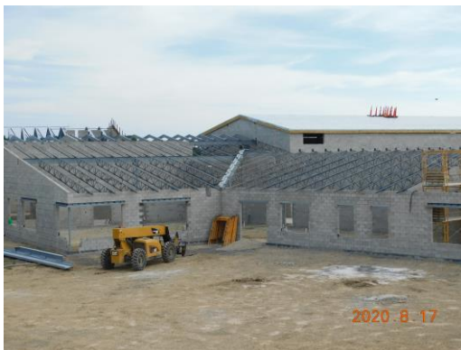
Steel being set over the Admin area
