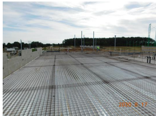
2 nd floor concrete prep with wire mesh is taking place
