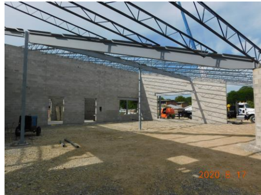
Steel installation in the media center
