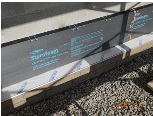
Unit A veneer, flashing and insulation has started
