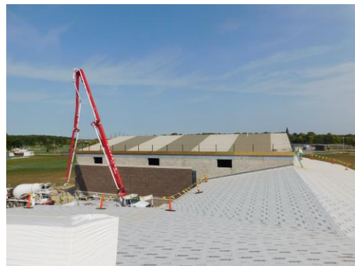
Day 2 gym roof pour completed last week
