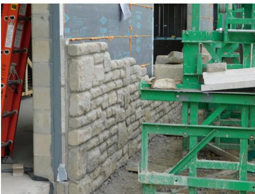
Stone being installed at the main entrance of the building
