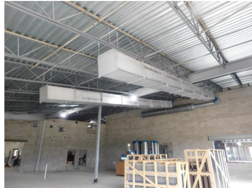
Ductwork has started in the media center
