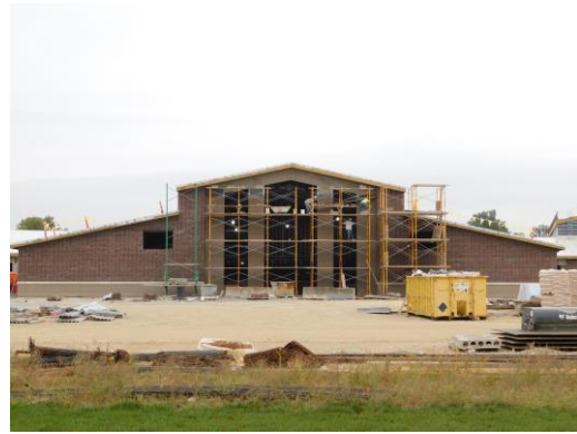
Veneer almost complete at the east side of the student dining
