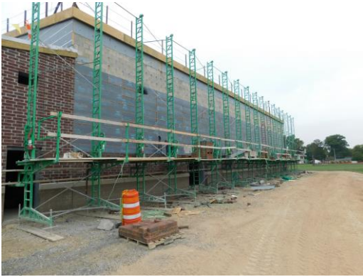
Veneer work taking place on the North side of the gym
