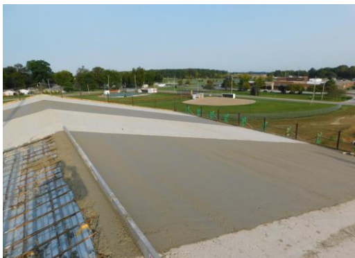
2 nd pour took place last week for the gym roof
