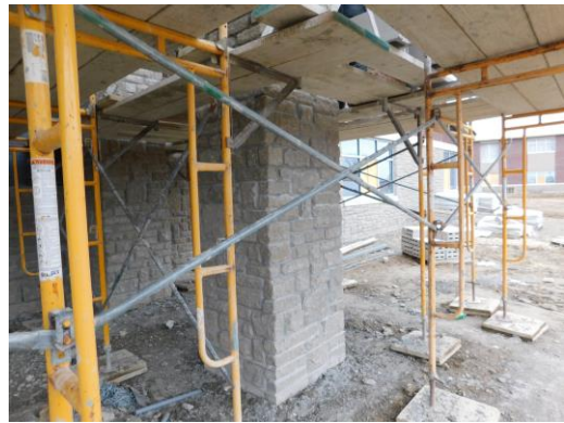
Cast stone veneer installation taking place at the main entry columns
