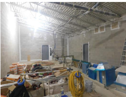
Main equipment room being prepped for block fill
