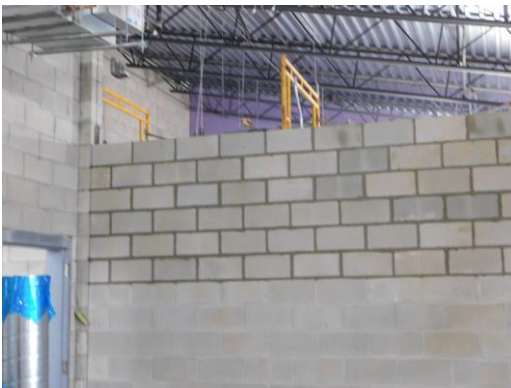
Interior CMU walls being installed on 2 nd floor
