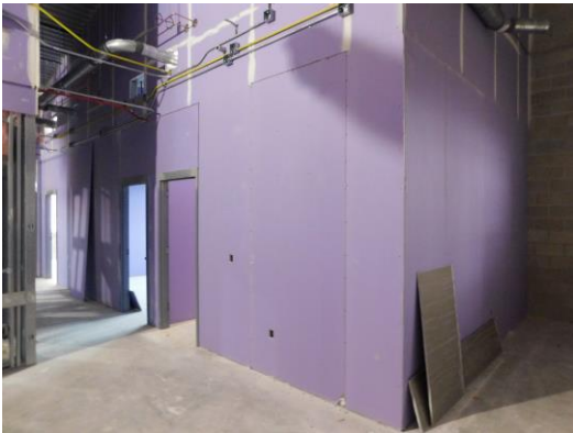
Drywall being installed in the admin area
