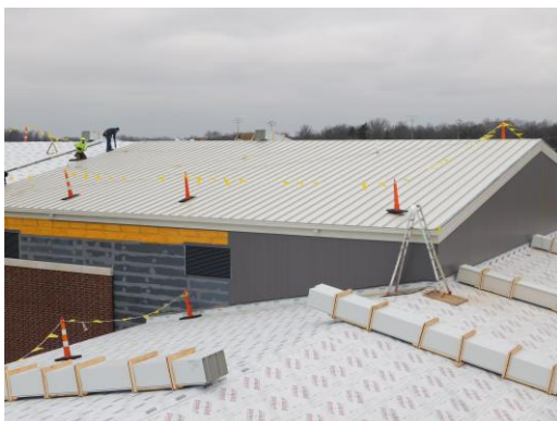
Metal roof panels being installed on the gym
